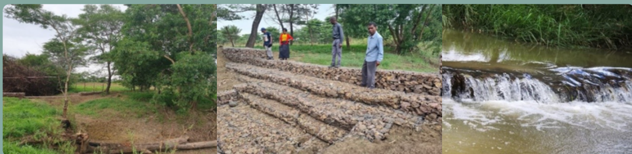
Construction of local check dam in Zambia: Courtesy RT Zambia
